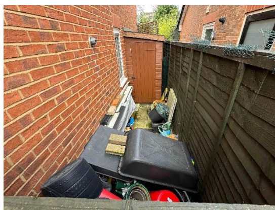
Stored items and shed restricted my inspection
