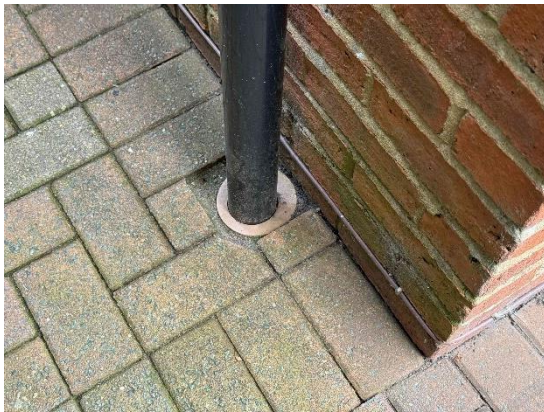
Downpipe pass below ground and are assumed to connect to a suitable discharge point such as a drain or soakaway
