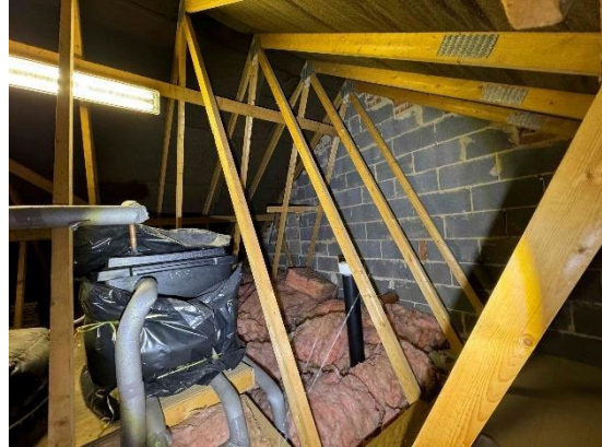
Roof void – main roof
