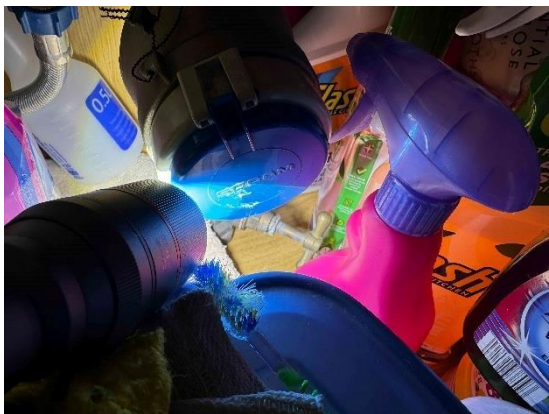
Internal stop tap - kitchen
