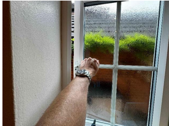
Windows checked for operation
