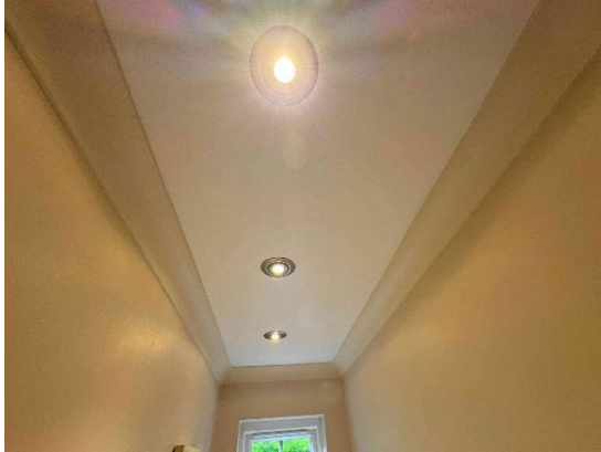
Modern plasterboard ceilings with plaster skim finishes
