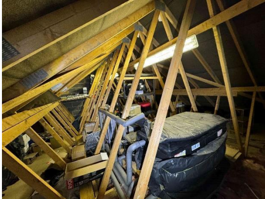
Roof void – main roof
