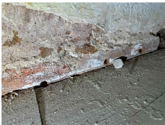
Remedial injected damp proof course
