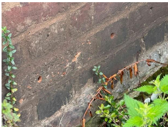
Remedial injected damp proof course
