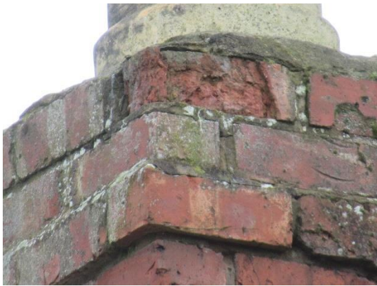
Weathered masonry
