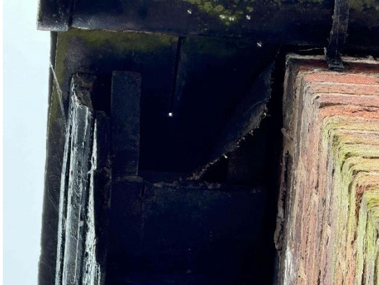
Underlay damaged
