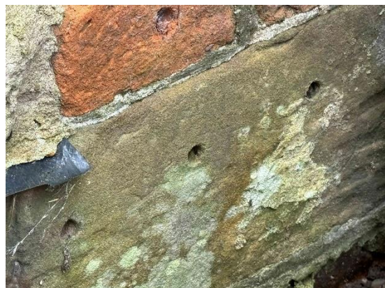
Remedial injected damp proof course
