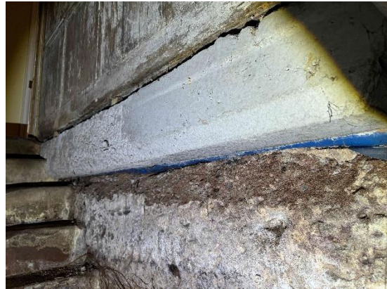
Evidence of new concrete floor with damp proof membrane
