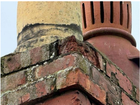
Weathered masonry
