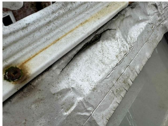
DIY self-adhesive repair with split
