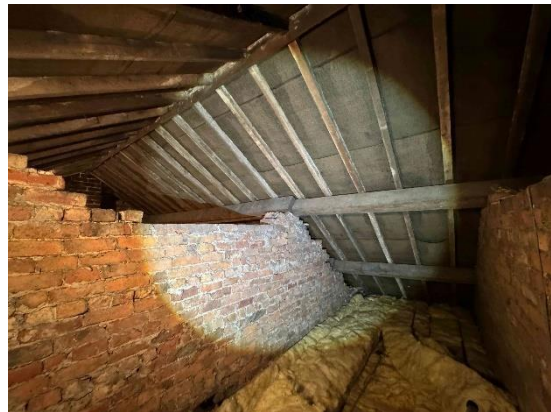
Main roof space / structure
