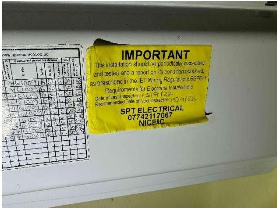
Sticker on the second consumer unit states that an inspection was carried out on the 15th September 2022, stating that another inspection should be carried out before 15th September 2032
