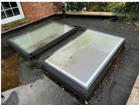
Rear extension roof
